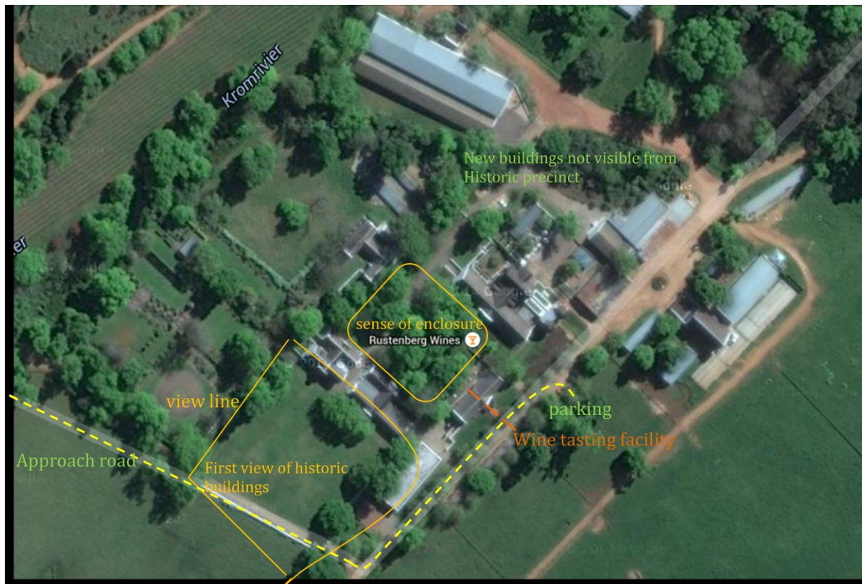
Figure 7: Google map view of the farm precinct showing the approach, the sudden exposure of the historic buildings, and the wine tasting facility situated at the side of the precinct (www.google maps).
